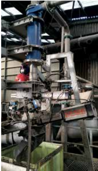
The Metamo degritter works with the Landia chopper pump to remove grit from the substrate before it goes to the digester
